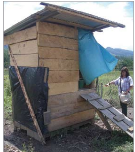
Caritas Project Coordinator, Rebeca, explains how the compost latrine works.
